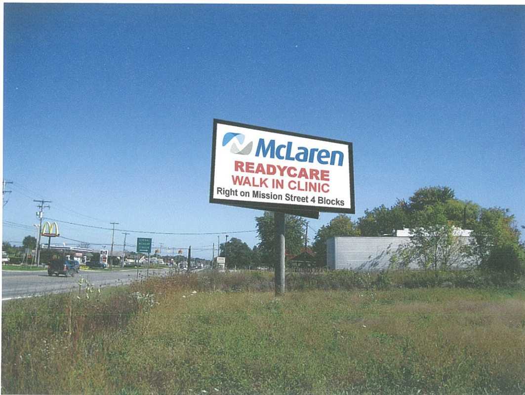
Install the existing sign 311 feet to the West
